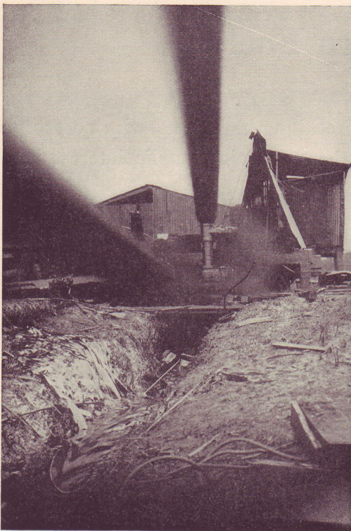
Valve half-way in place. As the heavy valve cut its way thru the column, the oil fanned out hundreds of feet to one side.
