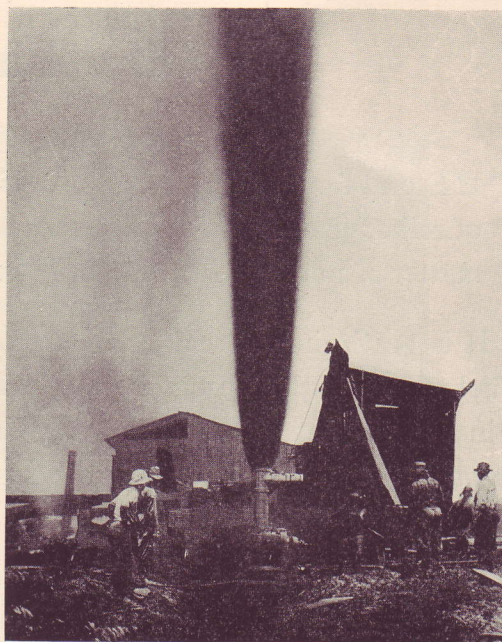
Valve on but open. When properly seated it was bolted down and the stem was lengthened thirty feet with a two inch pipe so that a man could get a safe distance from the well to close it in case of accident.
